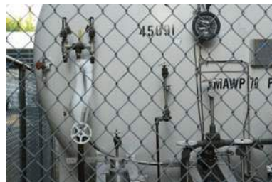
Difficult inspection sites
